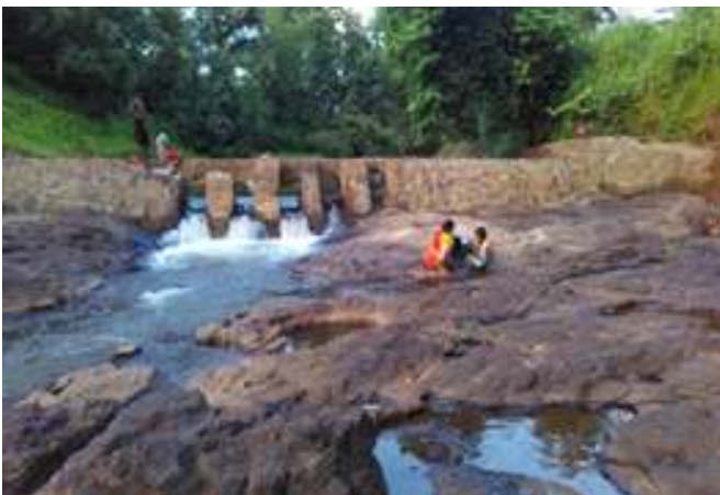
Bund with open vents
