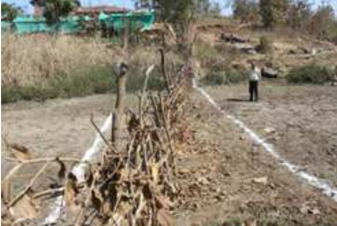
Pre bund construction site in Sonale
