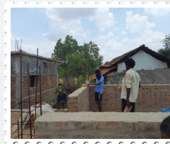
Eshwardas at a construction site
